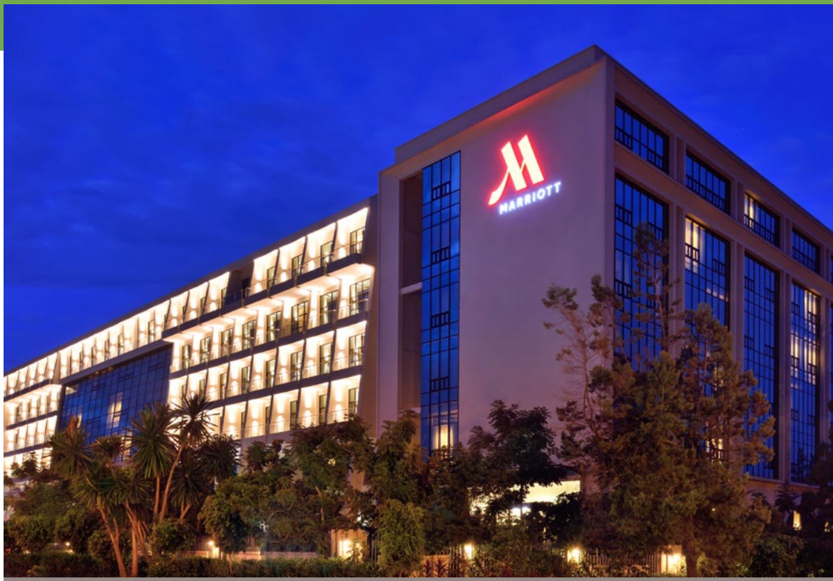
We opened our first Marriott hotel in Rwanda, the Marriott Kigali Hotel, in 2016.
